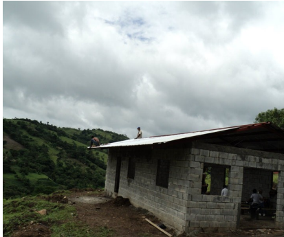
New Church Construction
